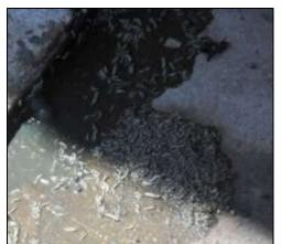
FIGURE 12 - Maggots and Leaking Sewage
